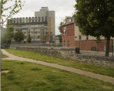
Grey wall copings were supplied piled to complement the colour of the natural stonework of the wall as well as the design, manufacture and installation of the steel railings. The total package was supplied by Procter Cast Stone.
